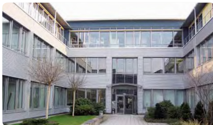
REICHENBACH- STRASSE 1 + 3, ISMANING
